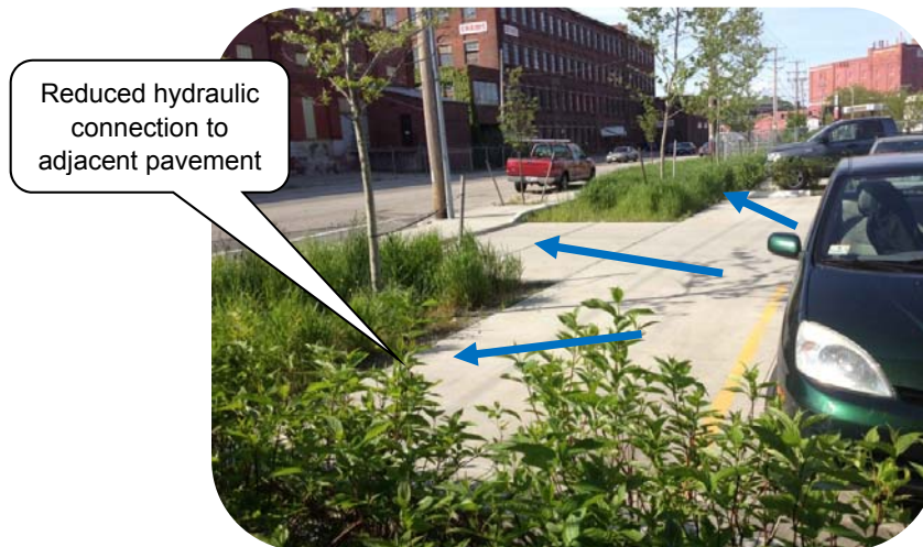
Example of Disconnecting Impervious Area from a Parking Lot in Providence, RI
