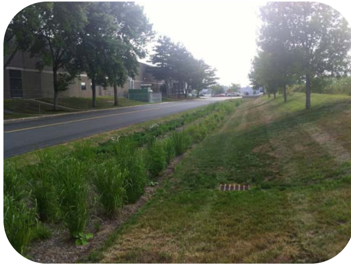
Underdrained Bioretention Swale, South Portland, Maine
