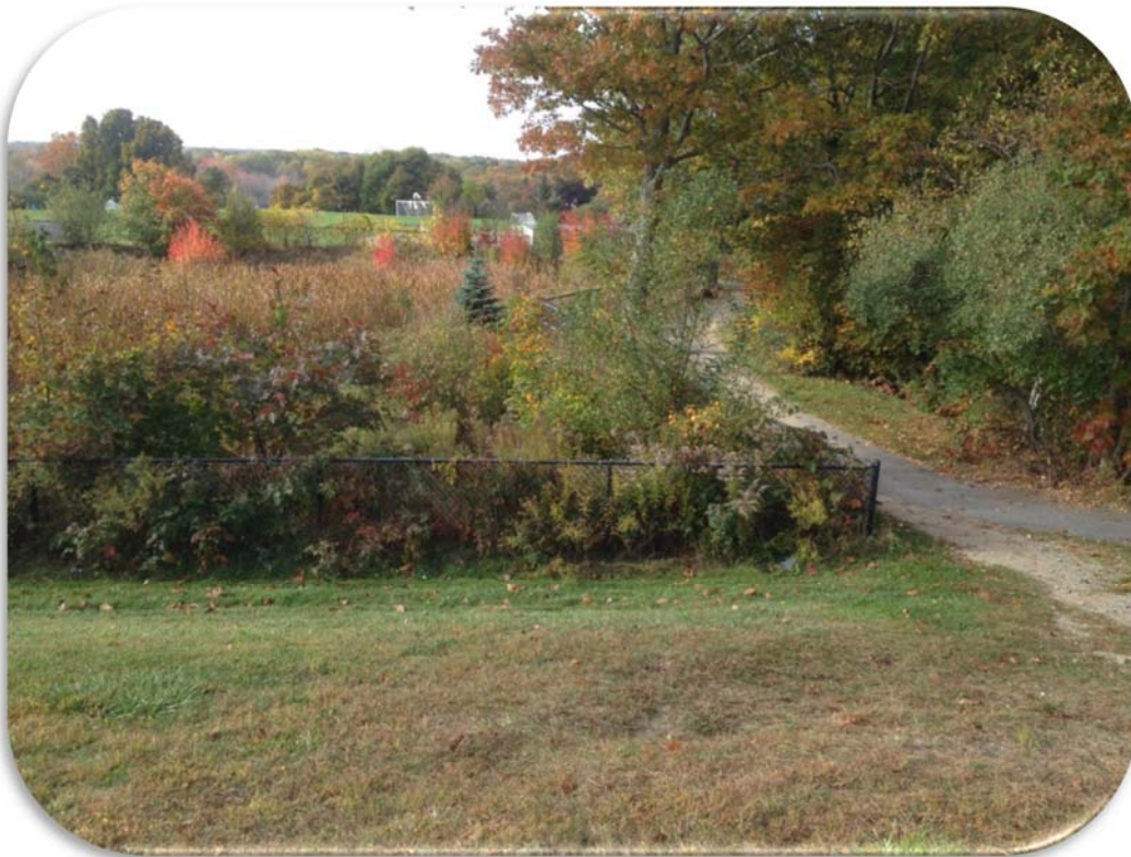
Detention Basin Adjacent to Softball Field (in background)
