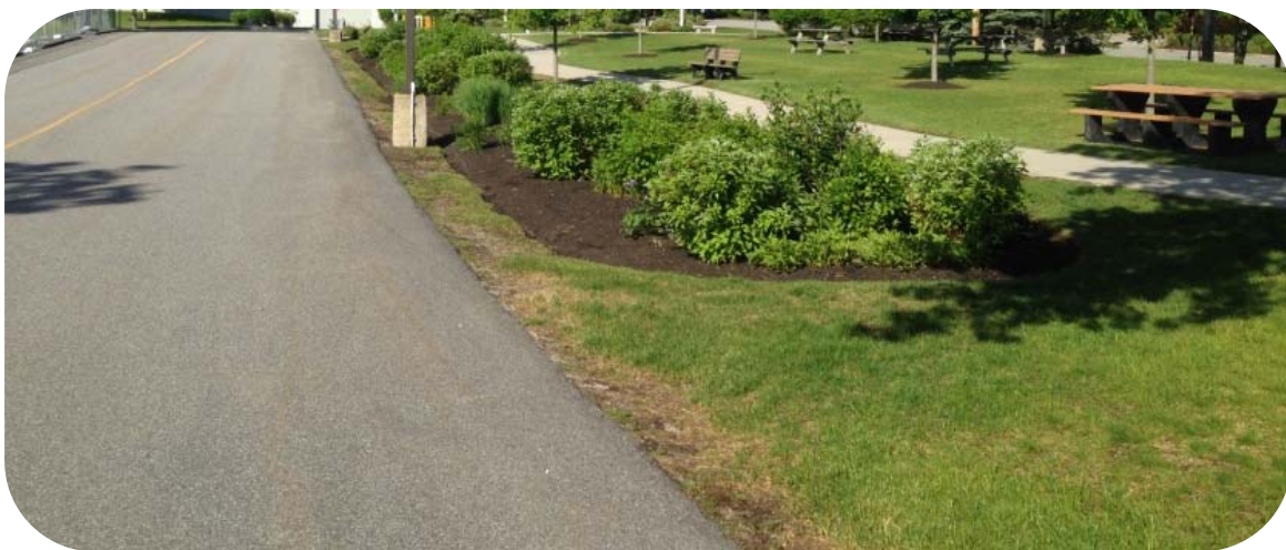
Bioretention Cell, South Portland, Maine
